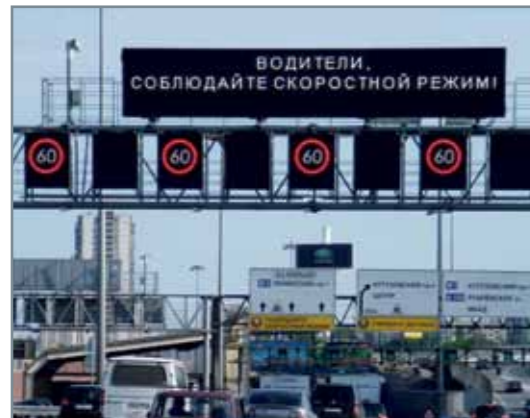
Freely programmable DRIP combination on a gantry with variable message signs showing limited content Russia
