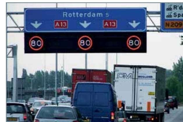
Signaalgever, limited variable message sign, 27 pictograms and 4 flashers The Netherlands
