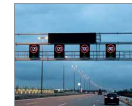
Limited variable message sign, speed limit with integrated lane control signaling
