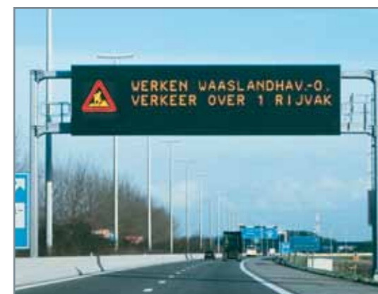
Full color, fully graphical, freely programmable RGB sign (left part) with freely programmable, fully graphical, yellow text area (right part) Belgium
