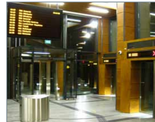
2-line and 10-line display, single sided, resolution 288x8 pixels/line, pixel pitch 4 and 6 mm, communication Ethernet, digital clock, cross&arrow sign
